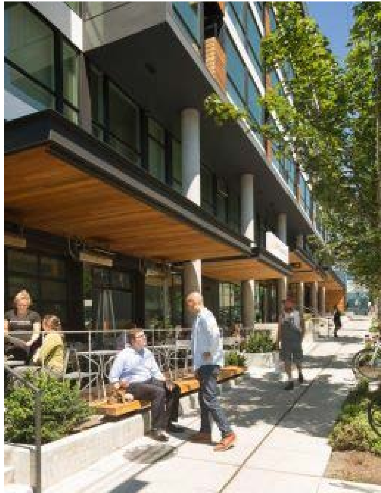
Ground floor designed using generously sized metal awnings
