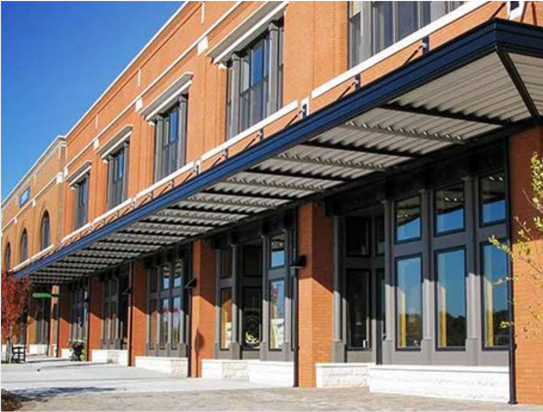
Example of generously sized awnings providing shade and preserving transparency
