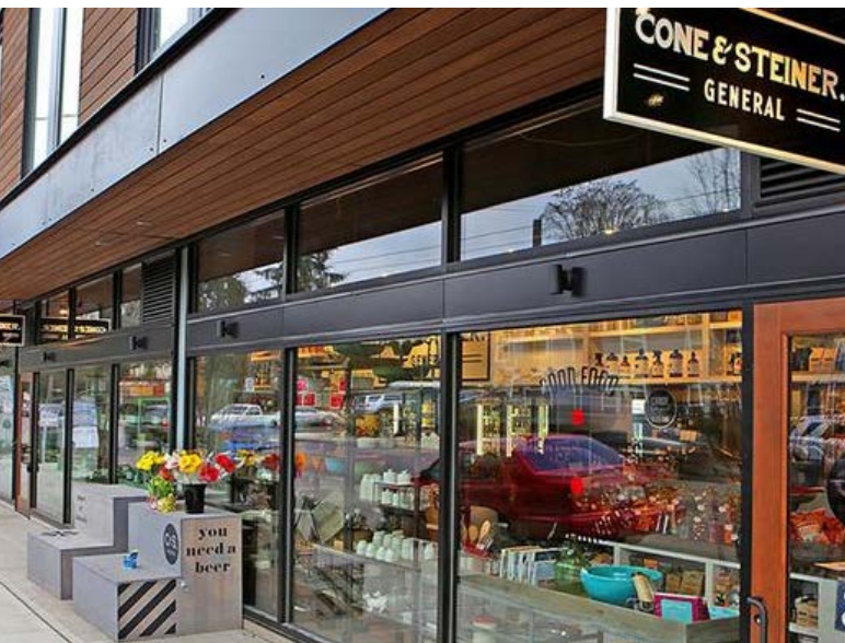
Transparency allowing views into retail shops and building uses
